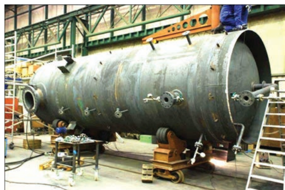
Figure 2. Submerged arc welding with cored wire: Austenitic CrNi steel AISI 310S
