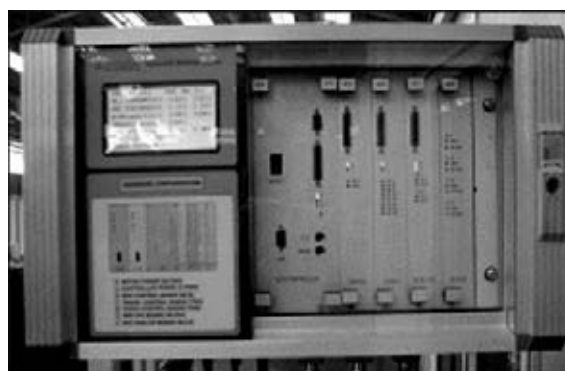
Figure 4. Main control unit
