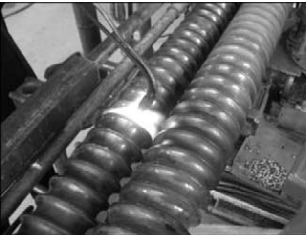
Figure 9. Performing circumferential non-closed heating
