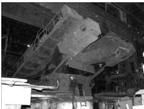
Figure 1. Tilted stand crosshead after wrecking
