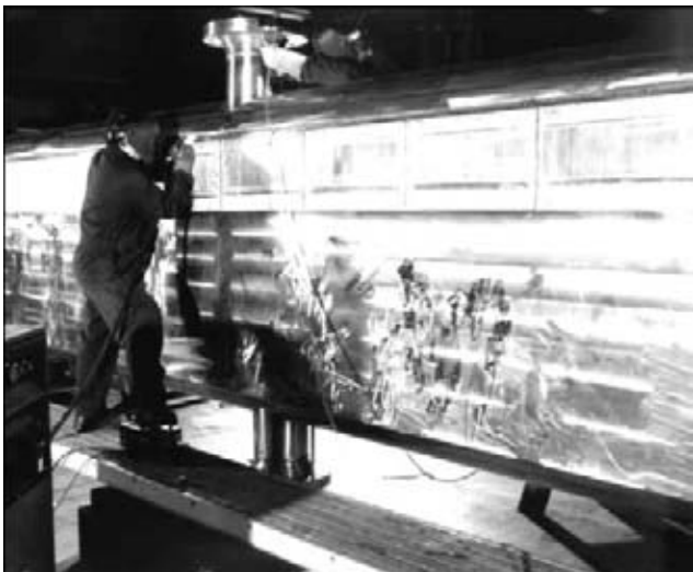
Figure 4. Welding headers to the exchanger core
