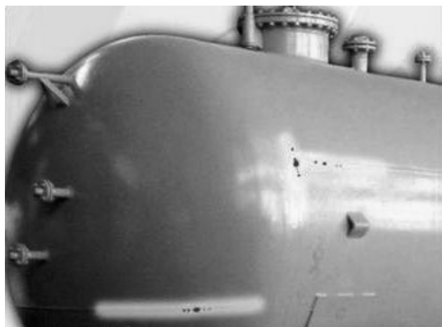
Fig. 4. Indication traces of leaks after chemical testing
