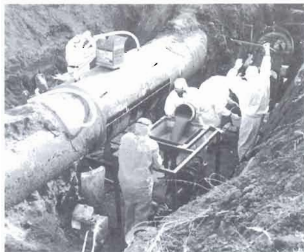
Figure 4. Filling the installed coupling with a composite compound
