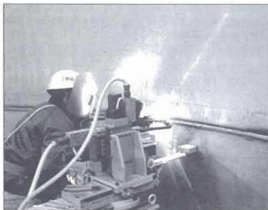
Figure 5. Detail of weld, arrangement of welding torch, magnetic coil and filler wire
