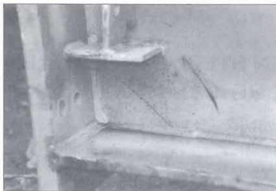
Figure 3. Crack in the web plate 18 mm thick between the cross-piece and flange
