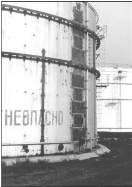
Figure 1. General view of a section of 20000 m 3 tank wall with special inserts used instead of a straight-line erection joint
