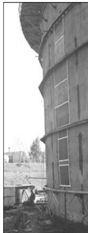
Figure 5. General view of the assembly butt joint after repair made by welding of special inserts into tank of the oil-pumping station «Lisichansk». The tank has a capacity of 50,000 m 3 and is equipped with a floating cover («Pridneprovskije Magistralnye Nefteprodvy»). Performer — «Bikor» Company
