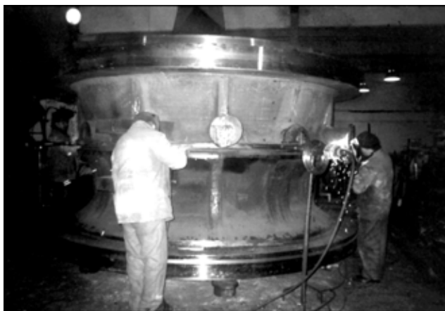
Figure 6. Welding of mill bowl
