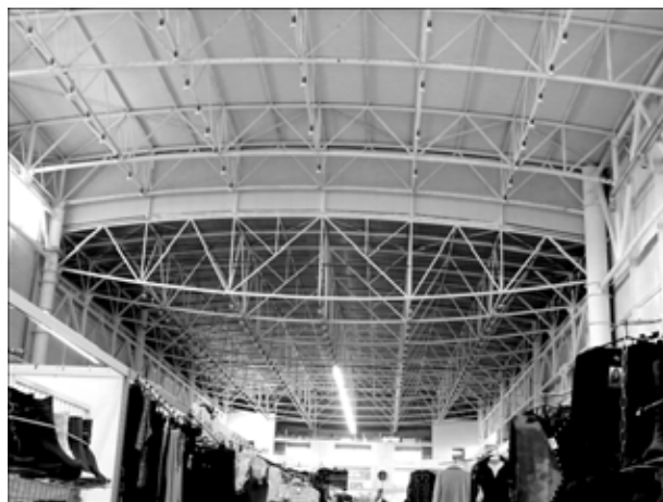
Figure 6. Tubular trusses of covering of the International Exhibition Center in Kiev
