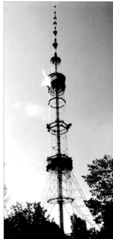
Figure 4. TV center tower in Kiev
