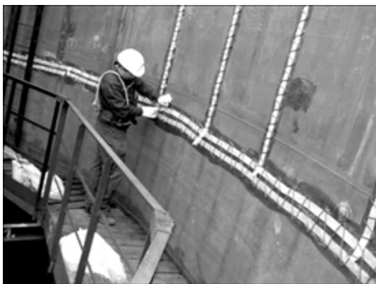
Figure 1. Mounting of explosive charge
