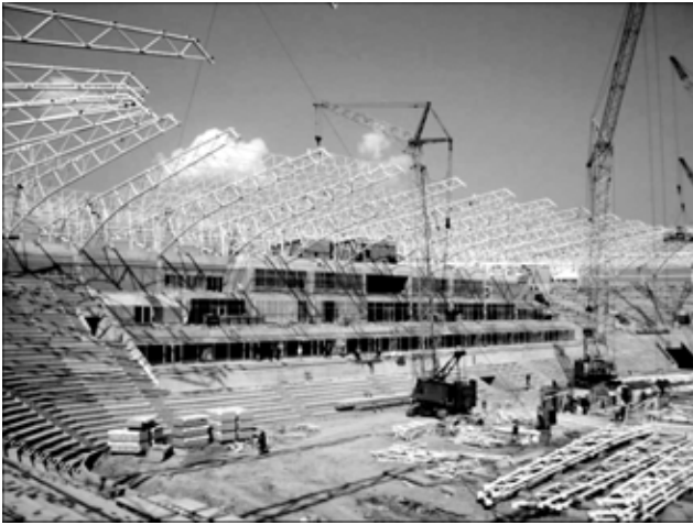
Figure 5. Mounting the stadium roofing in Dnepropetrovsk
