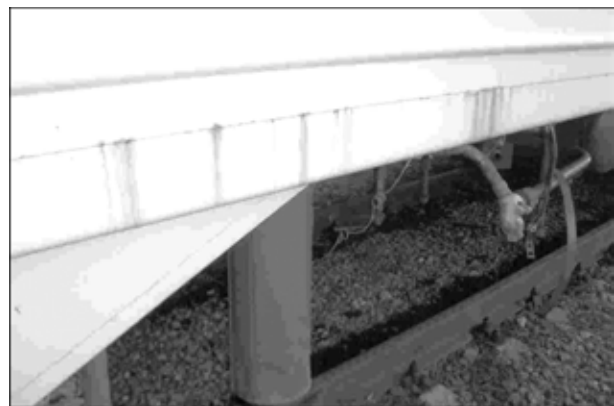
Figure 2. View of the carriage with weld defects developing during its service
