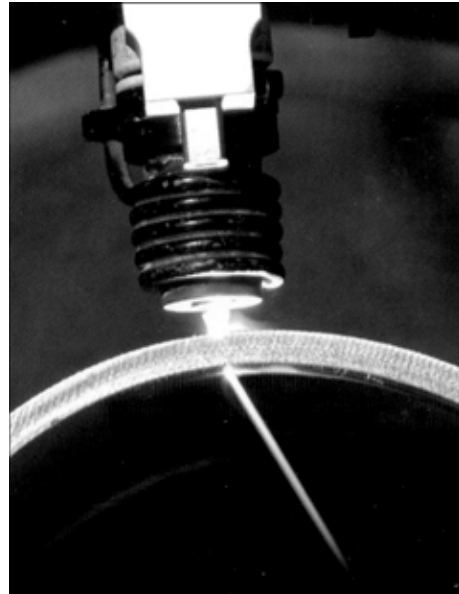
Figure 2. K-TIG welding of the pipe position butt joint 13 mm thick
