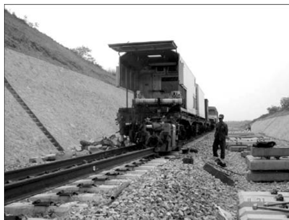
Figure 7. Welding of rails using K-922 mobile complex
