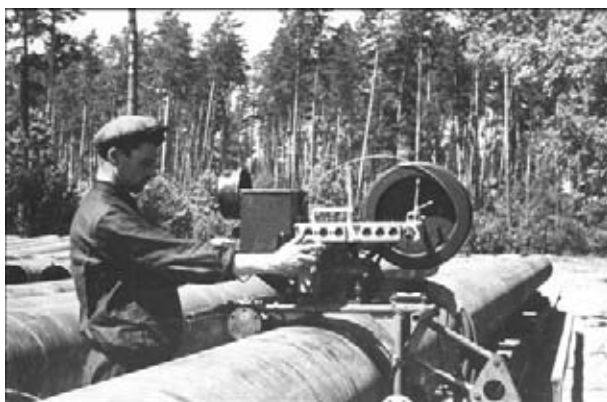
TS-17 in field camp of Dashava–Kiev gas pipeline
