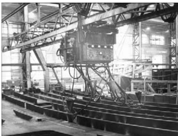
Mechanized submerged-arc welding of decking elements in Nikolaev Plant «Okean»
