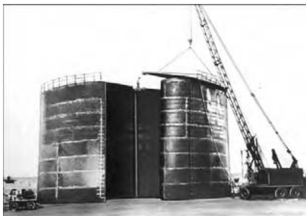
Mounting tanks of 10,000 m 3 capacity from coiled structures
