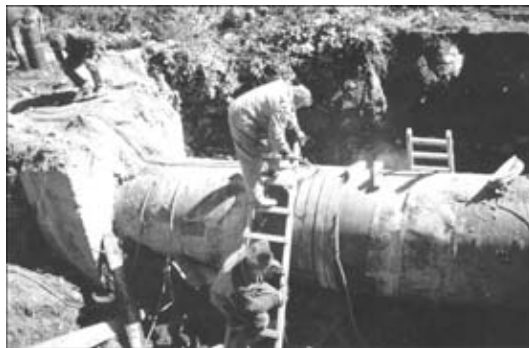
Assembly of overlap-butt joints on active pipeline
