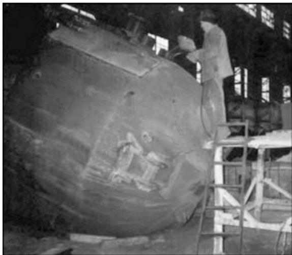
**Figure 6.** Repair welding of metallurgical equipment at the Dneprovsky F.E. Dzerzhinsky Metallurgical Works using the self-shielding flux-cored wire
