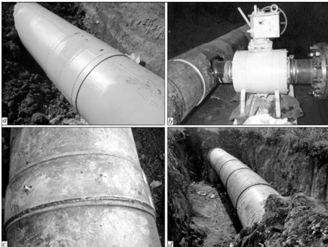
Figure 10. Mounting of sealed sleeve ( a ), branchpipe ( b ), two-layer sleeve ( c ) and bond-welded sleeves ( d ) on MP
