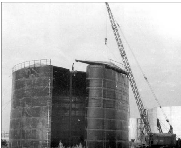
Erection of large-size tank (1948)
