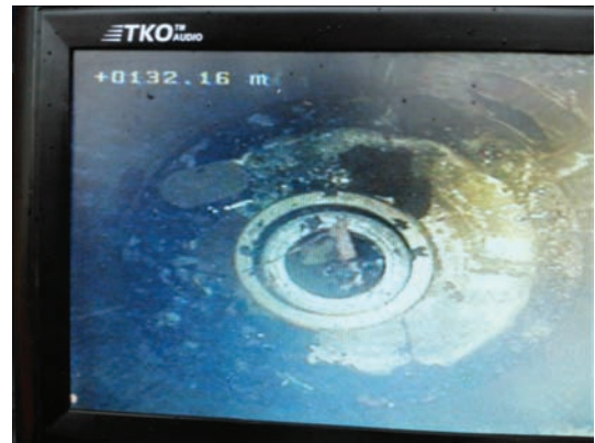
Figure 8. Appearance of welded-in bottom
