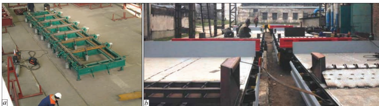
Figure 3. Typical objects of application of flux-cored wire welding: a — assembly-welding of frame of side wall of freight cars («Yugpromtekhmontazh» LLC, Kherson) [15]; b — welding of metal structures of platform for slabs, rails transporting («Verkhnedneprovsky machine-building plant» PJCS)
