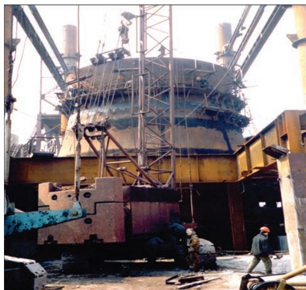
**Figure 7.** Repair of blast furnace DP-2 at the OJSC «Azovstal Steel Plant» using rolled steel 06G2B of the strength class C440. Welded metal structure with a total weight of 40 thous tons consists of 80 lower and facade columns with the length from 23 to 25.5 m, weight from 25 to 30 tons each, as well as beams of the lower and upper compressed rings (Figure 6).
