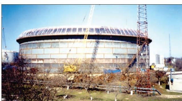
**Figure 4.** Tank for oil storage with a capacity of 75000 m<sup>3</sup> of rolled steel 06G2B-440
