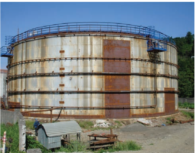
Tank with volume V = 10000\text{ m}^3 ( D = 34.2\text{ m} , H = 12.0\text{ m} ) for oil storage after repair
