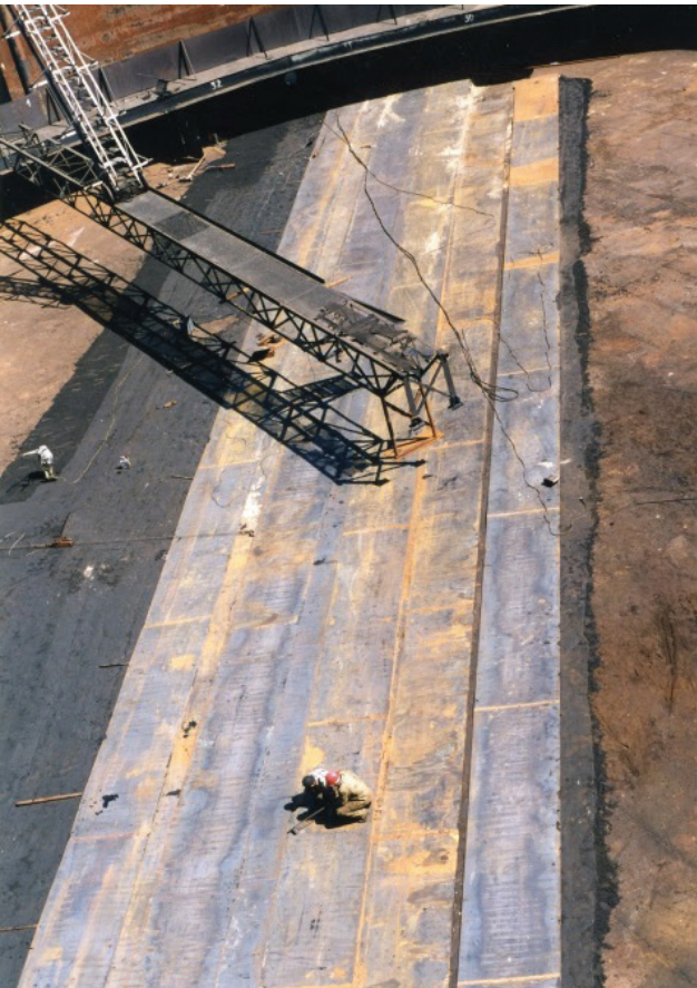
Tank with volume V = 50000\text{ m}^3 ( D = 60.7\text{ m} , H = 18.0\text{ m} ), replacement of the bottom and single deck of floating roof
