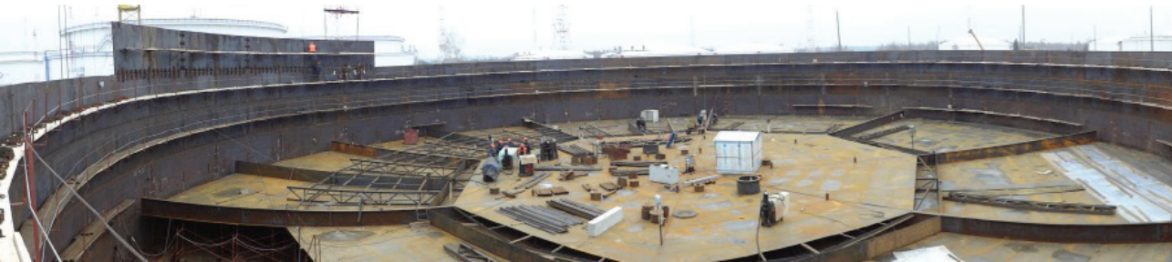
Tank with volume V = 50000 \text{ m}^3 ( D = 60.7 \text{ m} , H = 20.0 \text{ m} ) with double shell: erection the double deck steel floating roof
