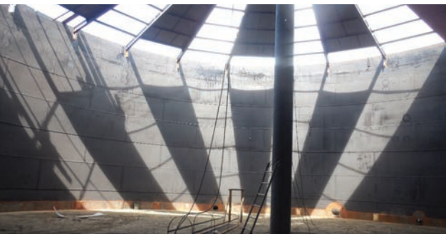
Repair of riveted tank with volume V = 5000\text{ m}^3 built in 1895 year
