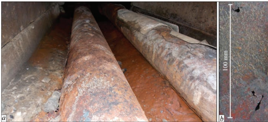
Figure 1. Feeding and return pipelines in a non-passable channel (a); through corrosion defects in the feeding pipeline (b)
