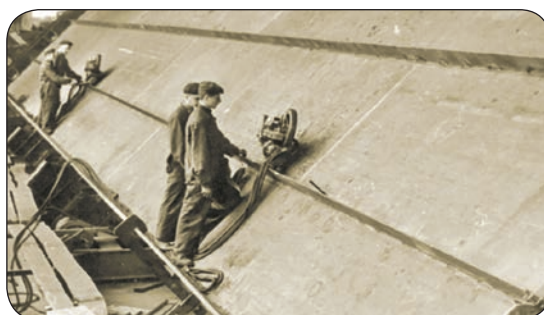
Welding of a bridge deck beam, Dnipropetrovsk, 1952
