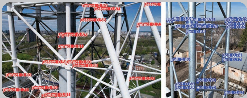
Detection results: AI-identified defects and bolts
