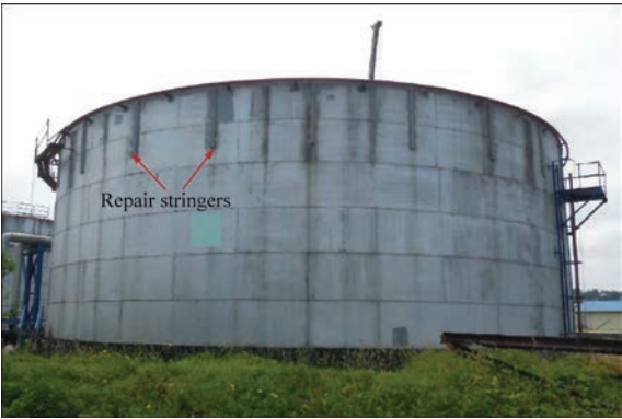
Figure 12. Repair stringers installed at the points where the radial beams are connected to the shell
