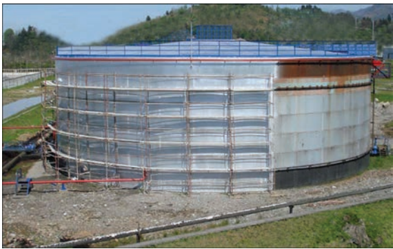
Figure 19. View of the tank, 1929 year, after repair during the application of an anti-corrosion coating
