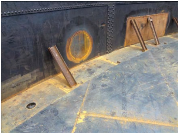
Figure 16. Installation of a new bottom: annular bottom plates of 8 mm thick, central part of 6 mm thick
