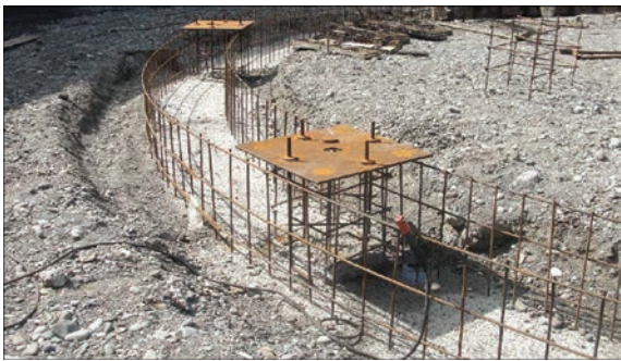
Figure 15. Installation of a reinforced concrete circular foundation for the supporting columns of the roof
