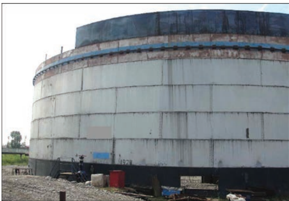
Figure 17. Replacement of the upper shell course with mounting of a fixing ring
