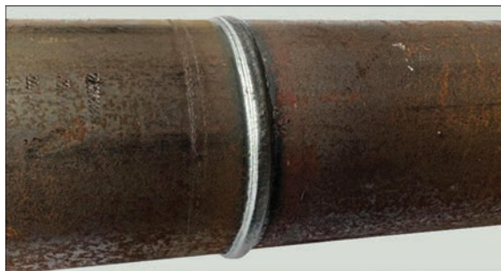
Figure 9. Technologically reduced weld reinforcement height on the pipe
