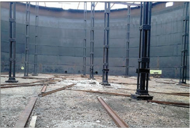
Figure 13. Dismantling of the existing bottom and roof of the tank, 1929 year
