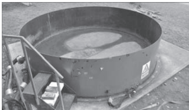
Figure 1. Tank floor of 4 m diameter
