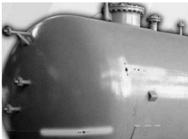
Fig. 4. Indication traces of leaks after chemical testing
