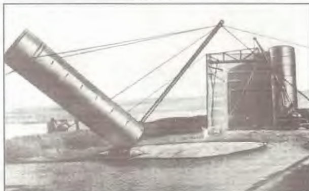
Erection of a large-sized tank (1948)
