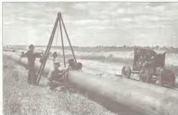
Automatic welding of pipeline in Dashava-Kyiv route (1949)
