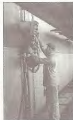
Automatic welding of vertical welds with a forced formation in the bridge span (1952)
