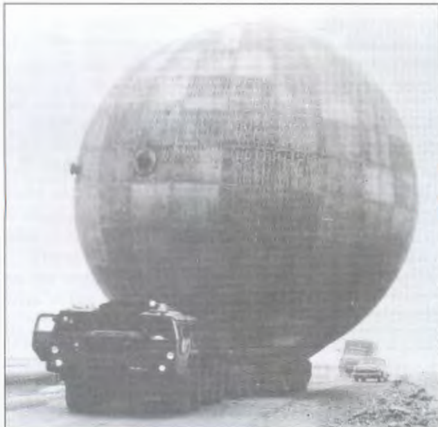
Figure 7. Transportation of the internal casting of the tank 110 t in weight to the erection site
