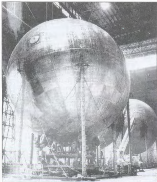
Figure 6. Automatic welding of the cryogenic vessel on a manipulator
