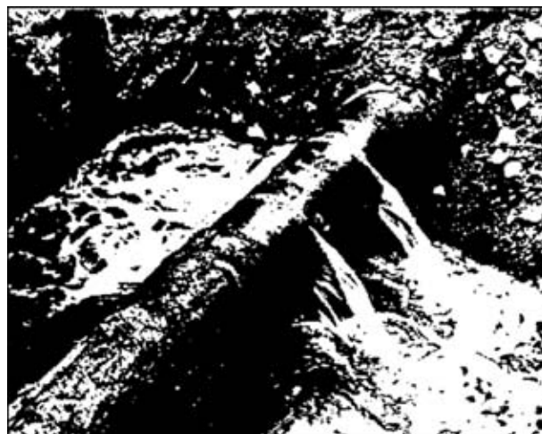
Figure 4. Outflow of petrol from pipeline after explosion cutting using foam protection
