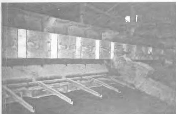
Figure 9. Aluminium contact pads for fastening electrolyzer anodes welded with PSh-107VA semi-automatic machines
