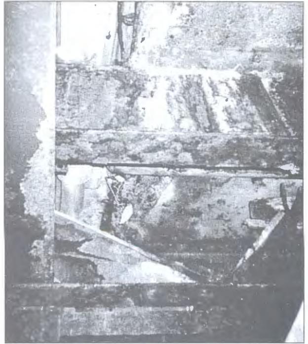
Figure 3. Appearance of corrosion failure of transversal beams in the E.O. Paton bridge
