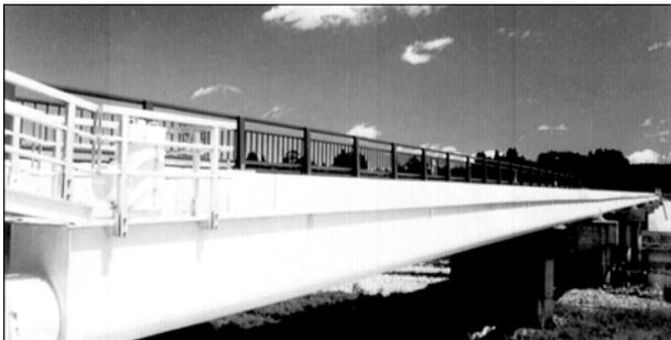
**Figure 1.** Overpass in Japan with aluminium metallised coating painted with acryl paint in two layers (coating service life is more than 25 years)
