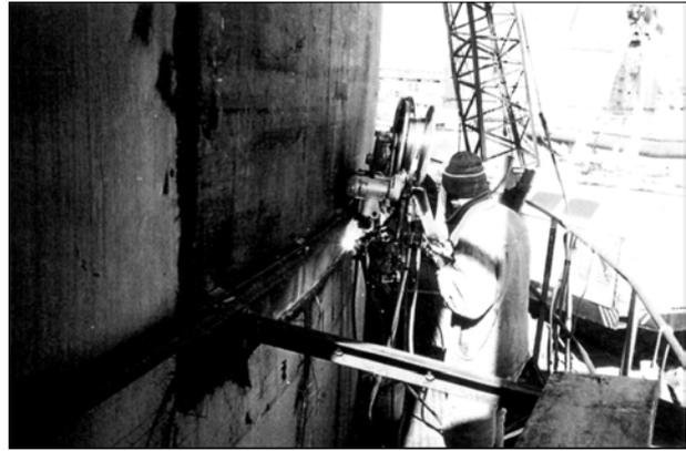
**Figure 3.** Automatic welding of a horizontal weld on a tank wall by AD-330M machine
