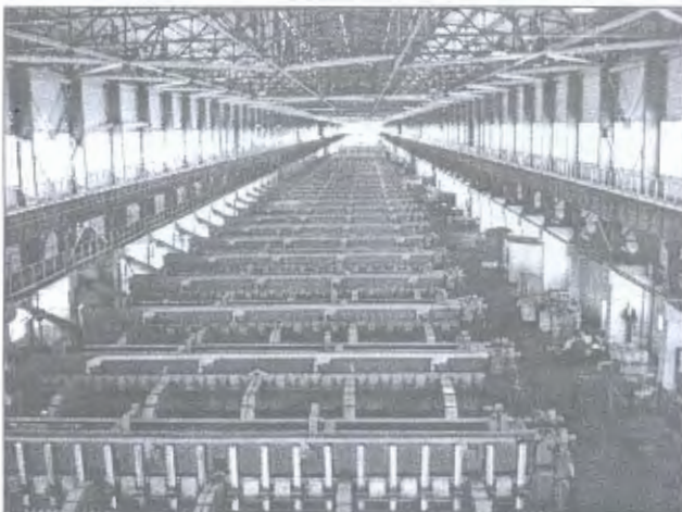
Figure 1. Shop No. 9 of Irkutsk Aluminium Plant under construction
