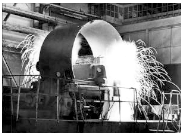
Flash butt welding of shells using machine K767
