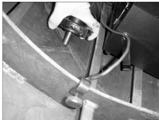
Figure 4. EDT of welded joints of stern strengthening of TC hull
