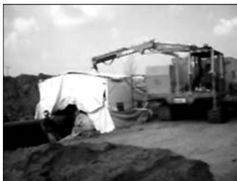
Figure 2. Building site in pipeline construction
