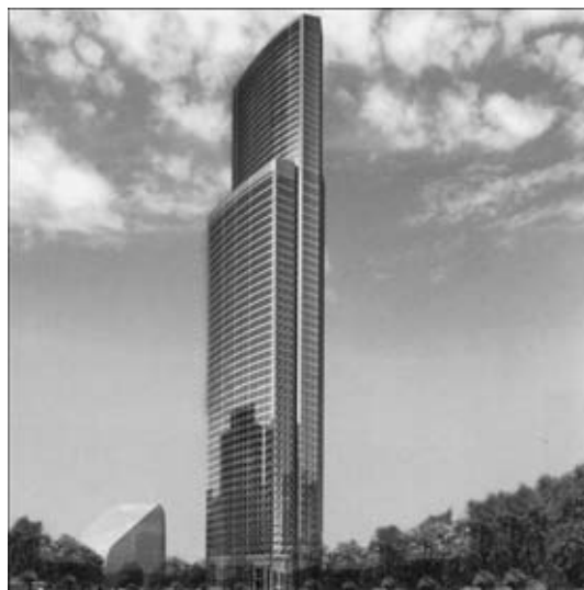
Figure 1. High-rise building «Eurasia» in Moscow
