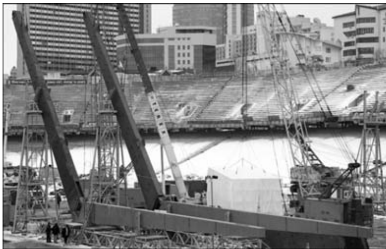
Figure 3. Appearance of columns ready for erection
