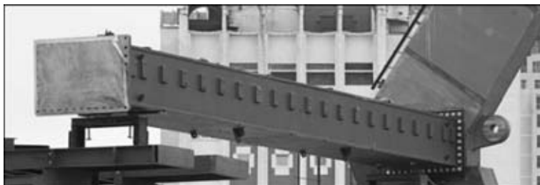
Figure 2. Compressed girth element in site
