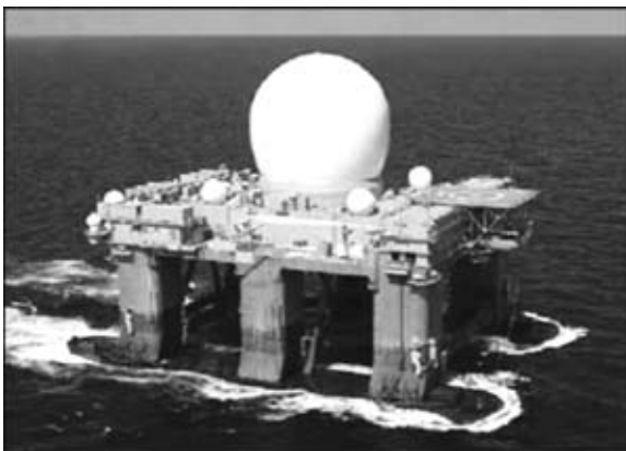
Figure 6. Air-supported structure of radome on ILC Dover testing platform in the Gulf of Mexico [6]
