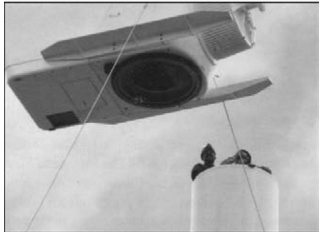
**Figure 3.** Mounting a powerful wind generator nacelle on wind generator tower
