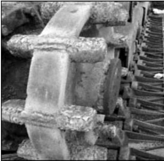
Figure 4. Appearance of repaired drive sprocket of crane KS8165
