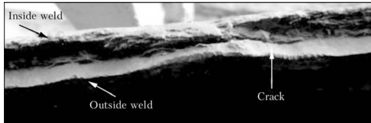
Figure 2. Crack in outside longitudinal weld on failed pipe of 820 mm diameter
