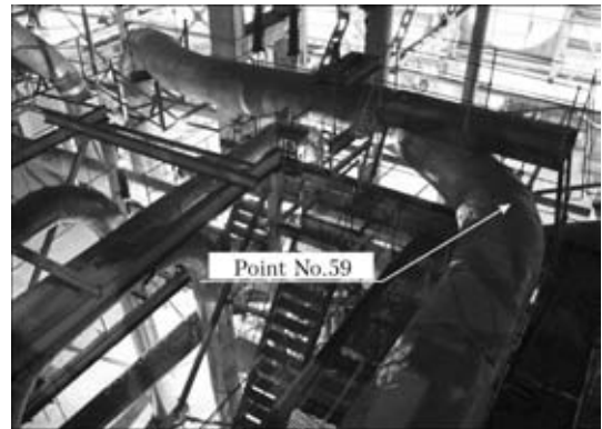
Figure 19. One of points of measurement by AE of operation activity of pipeline of steam intermediate overheating at Kiev HES-6
