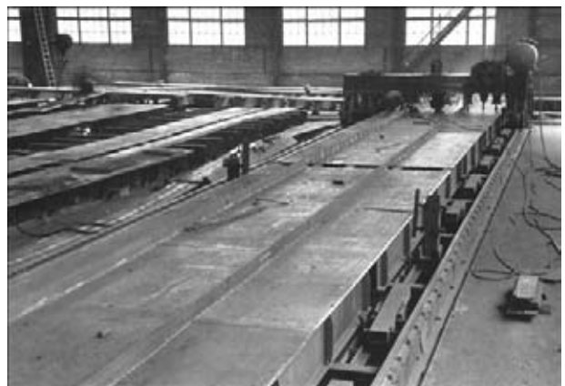
Figure 3. Process of assembly of trusses in the rig
