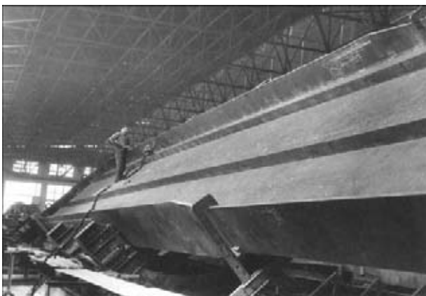
Figure 7. Process of welding of longitudinal butts using tractor TS-17M in the tilter
