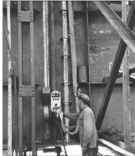
Figure 13. Welding of vertical site butt using automatic machine A-314
