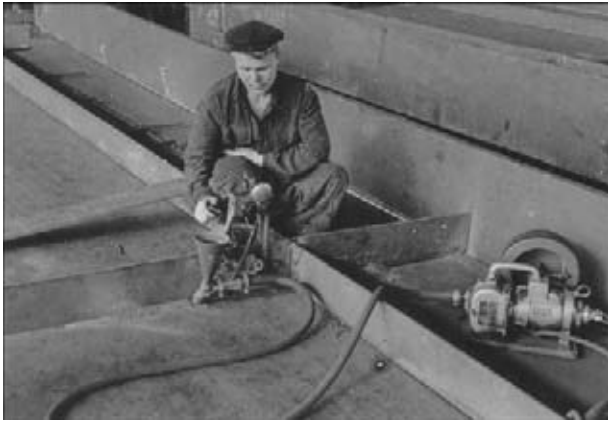
Figure 6. Welding-on of stiffener using semi-automatic machine PSh-5 with holder DSh-27
