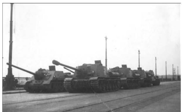
Figure 15. Testing of the bridge
