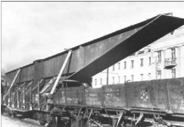
Figure 12. Haunch loaded on the platform
