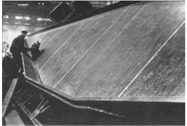
Figure 9. Welding of girth welds of haunch in the rig
