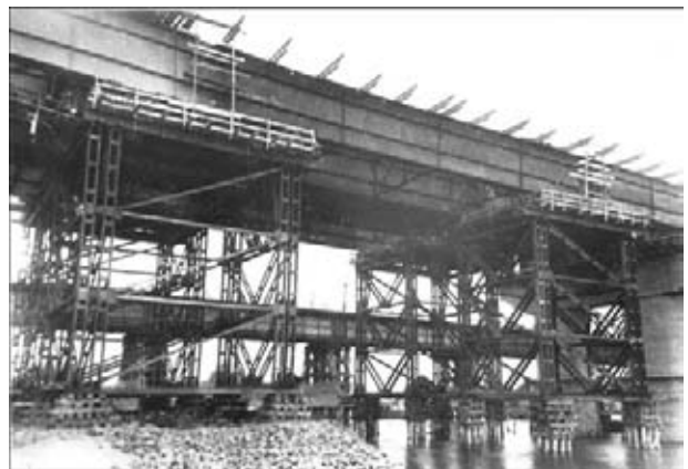
Figure 14. General view of welded site butt in the span
