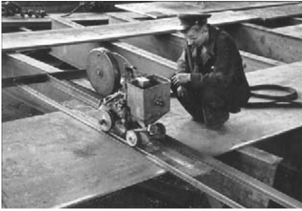
Figure 5. Welding of wall butt weld using tractor TS-17-M
