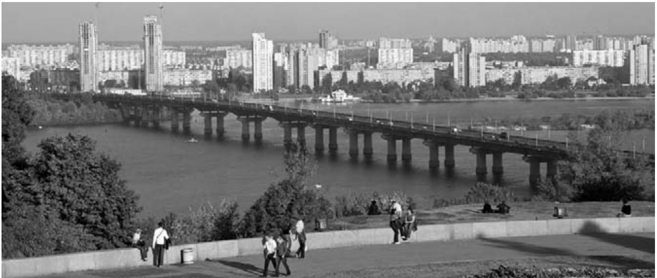
Figure 1. All-welded E.O. Paton bridge across the Dnieper river in Kiev
