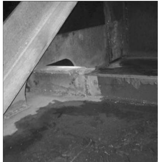
Figure 6. Welded assembly of modified design
