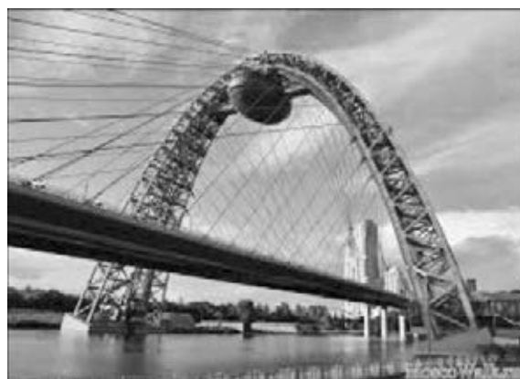
Figure 6. Bridge crossing in Serebryany Bor (Moscow)
