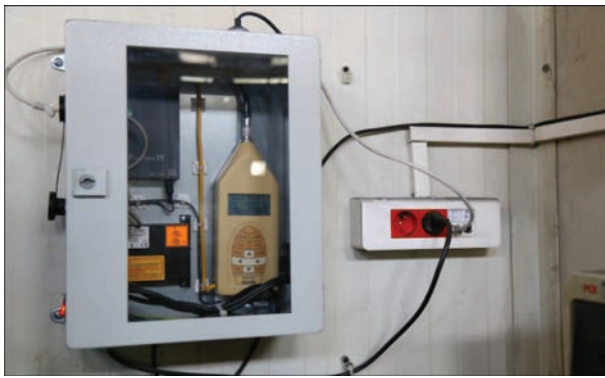
Figure 3. Noise meter in the production floor
