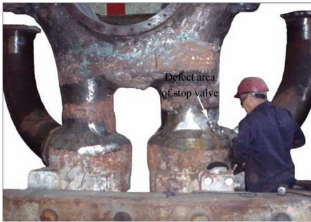
Figure 2. MPC cover with stop valves during preparation for repair
