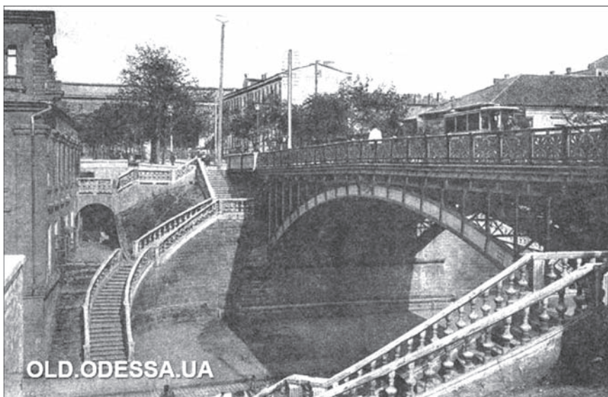
Figure 1. General view of the bridge at the end of the XIX century
