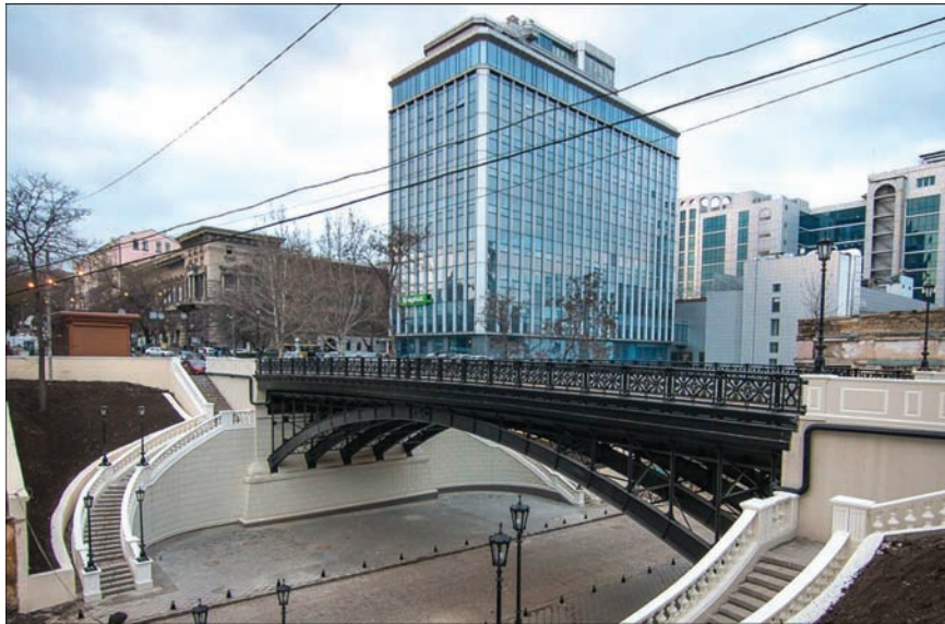
Figure 7. General view of the reconstructed bridge with the restored architectural and decorative railing elements (November, 2017)
