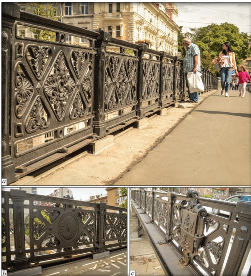
Figure 6. General view of railing ensemble (August-September 2017): a — appearance of renovated panel of railing grates; b — under emblem grate with emblem (view from the sidewalk); c — view from the outside of the bridge
