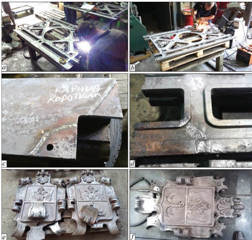
Figure 5. Fragments of restoration works: a — restoration of under emblem grate by welding; b — final cleaning of welds; c — type of repaired joint on short cornice; d — type of repaired joint on grate No. 13; e — type of emblems before restoration (in the foreground, newly cast fragments of lost decorations — volutes); f — type of emblem No. 1 after restoration
